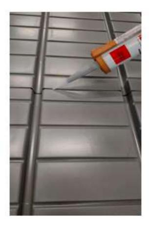
STEP 1: Lay trays out per included drawing. Trays should have roughly a 1/8" Gap, There is a planned air gap in the end to allow for expansion. Make sure all trays are sitting level before moving on to the next step.
