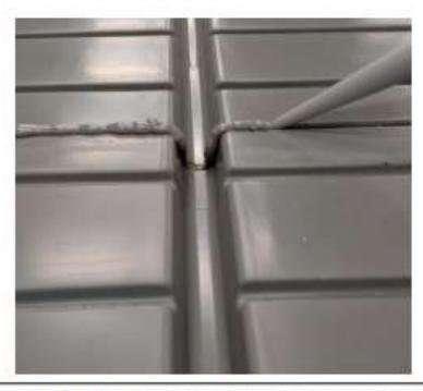
Step 3: Run a bead of glue filling up the 1/8" gap you left, allow extra to run down the main drainage channel. Use a small utensils such as a small piece of plastic or metal pipe to smooth glue in main drainage channel, Making sure there is a seam sealed on both ends and no large globs blocking water flowage. You may have to repeat this 1 or 2 times after a few minutes. DO NOT Smooth glue on the top of the gap, let it settle by gravity only smooth glue in the drainage channel.
